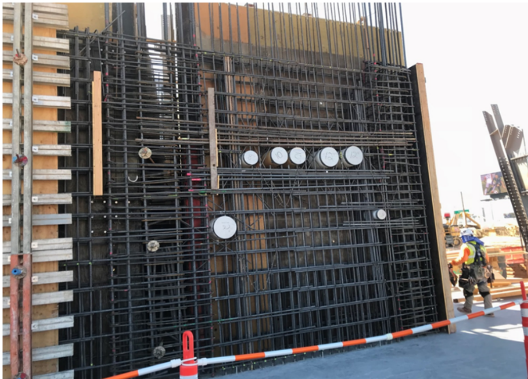
Rebar and Form work continues in the Cores
