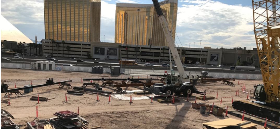
Steel truss column assembly beginning on site.
